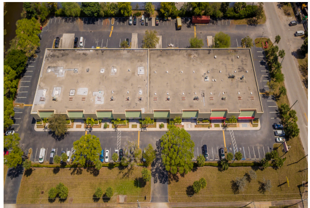
Aerial View - Powerline Road Frontage
