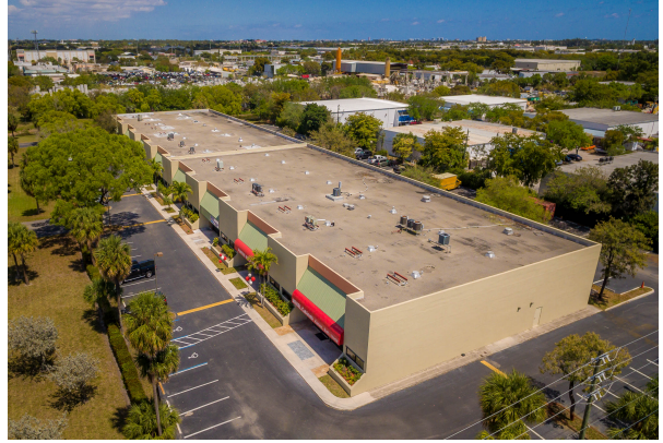
Aerial View - Building Frontage
